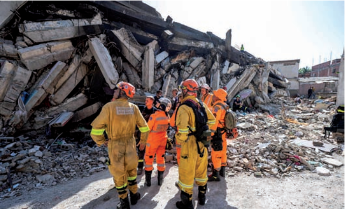
Rescue workers trying to find a way inside a damaged building in, Venezuela, yesterday. (AFP)
