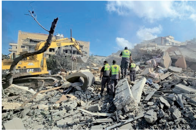
Civil defence workers search through the rubble following an Israeli strike in the southern Lebanese area of Al-Hosh yesterday. (AFP)
