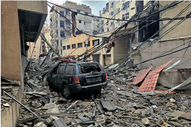
Debris is strewn along a street and after a residential apartment block was struck in an Israeli airstrike in Beirut's southern suburb of Haret Hreik yesterday. (AFP)
