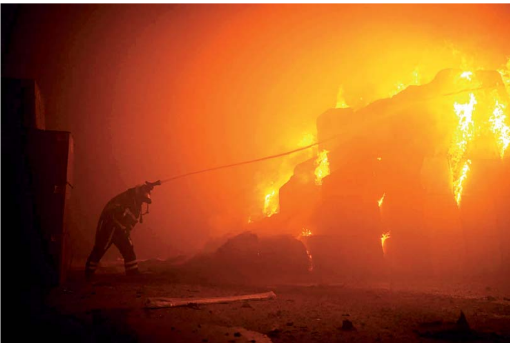
A rescuer putting out a fire in a building, as a result of falling debris after a massive drone attack mainly targeting the Ukrainian capital, in Kiev. (AFP)
