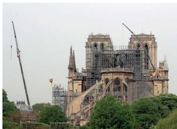
Workers install temporary tarpaulins to protect Notre-Dame Cathedral from rain, in Paris, yesterday.
